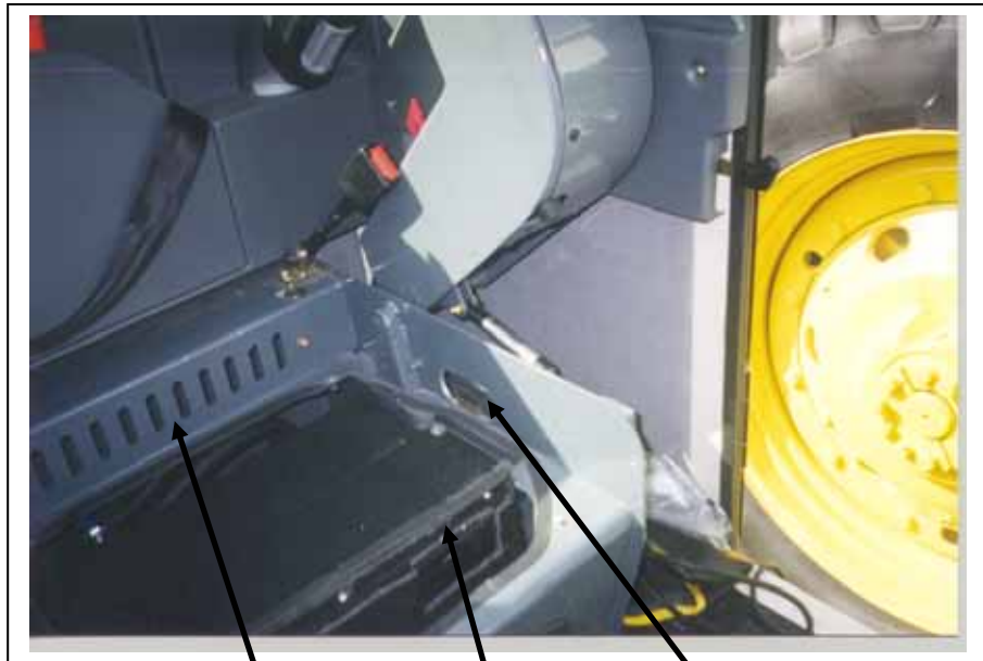
Inside air panel removed
